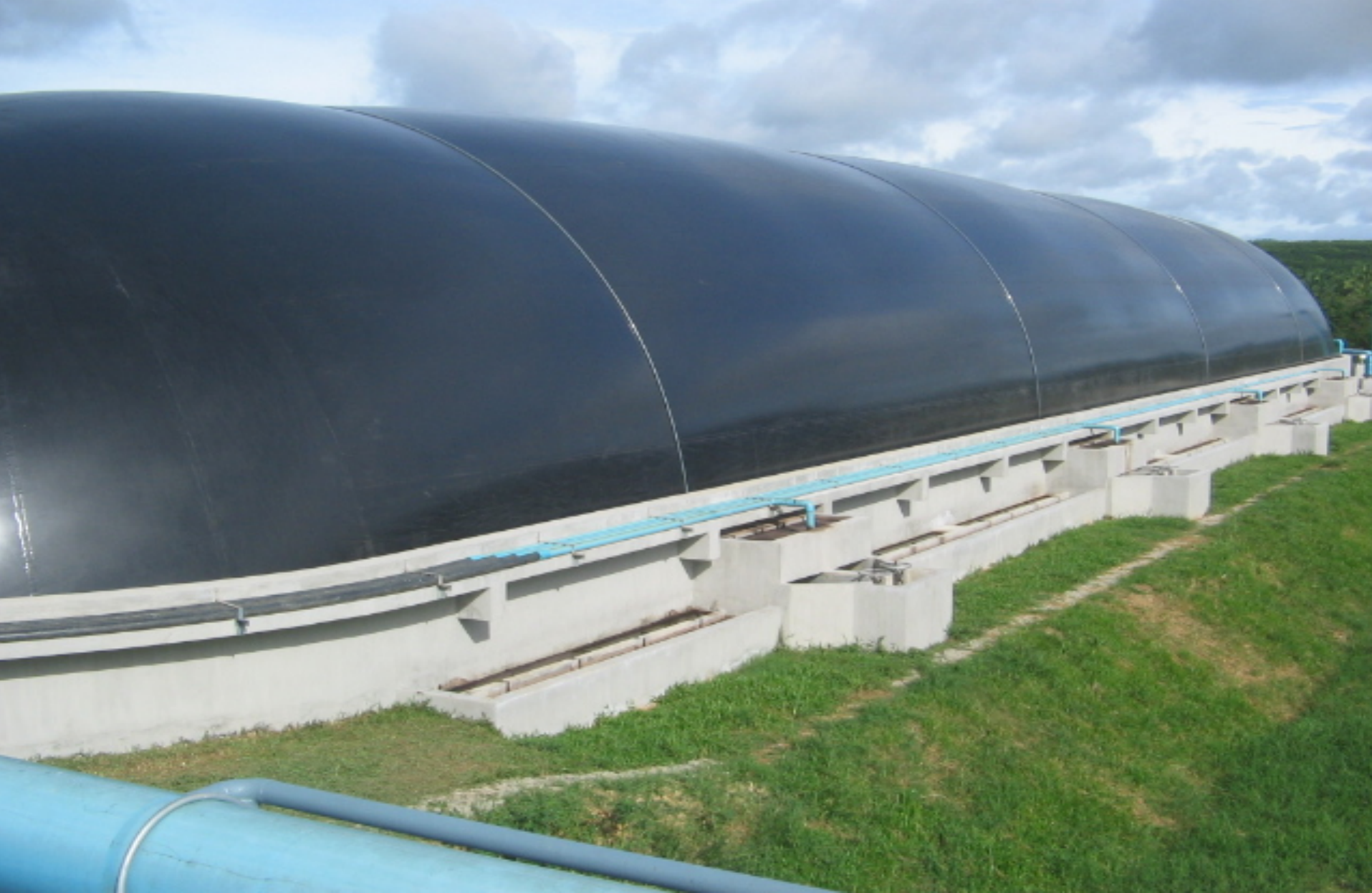
Appropriate + Complete Stirred Tank, Thailand (A+CSTRTh) Reactor
