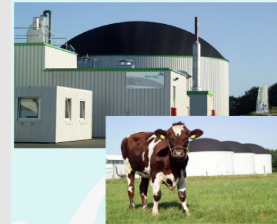
© Schmack Biogas AG
