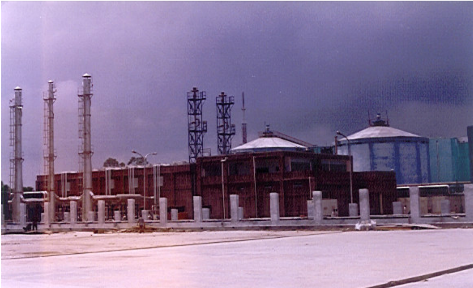
Project for generation of 5 MW power from Municipal Solid Waste at Lucknow (courtesy MNRE)
