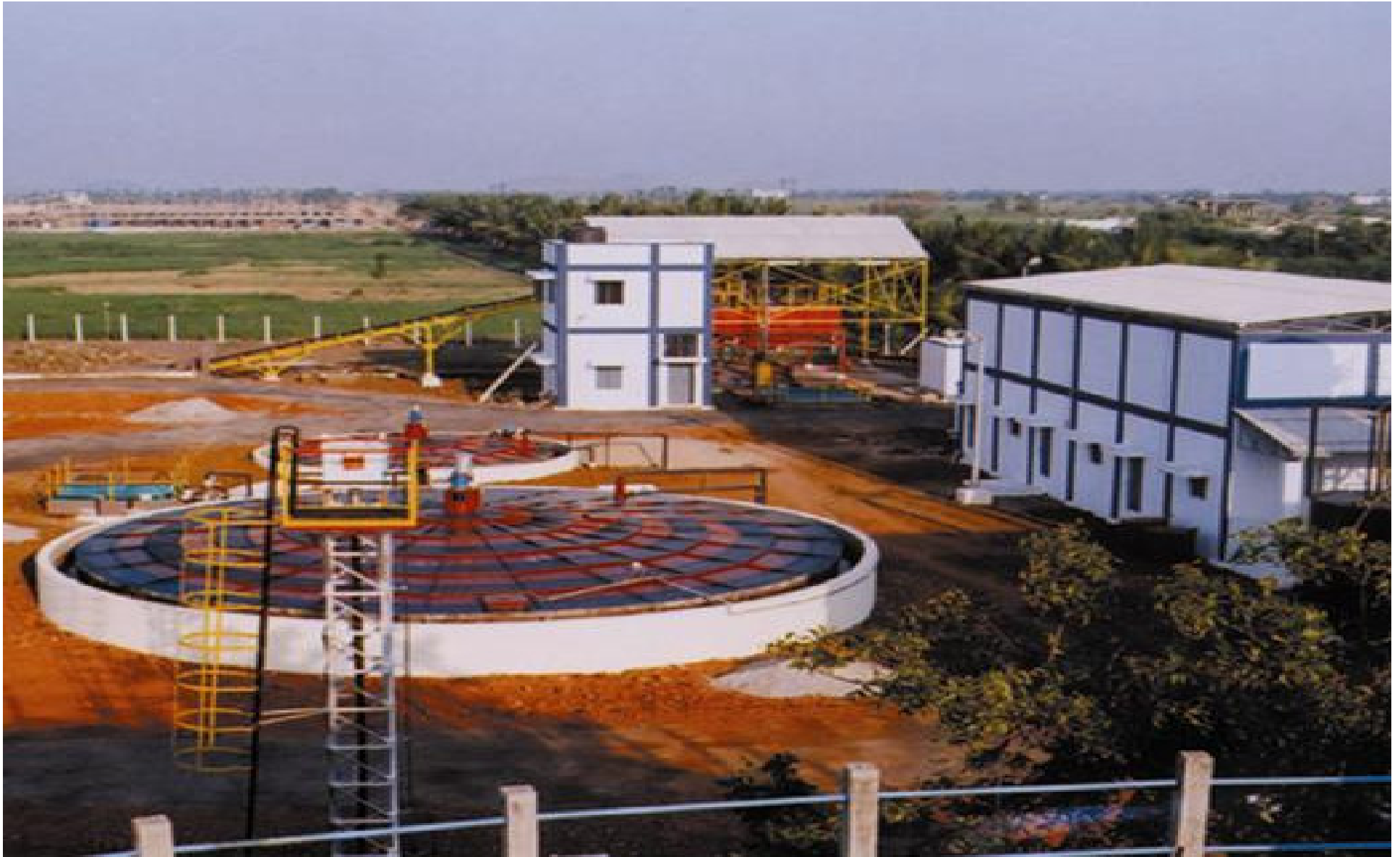
0.15 MW Power Project Utilizing Vegetable Market and Slaughterhouse Wastes at Vijayawada, A.P. (courtesy MNRE)
