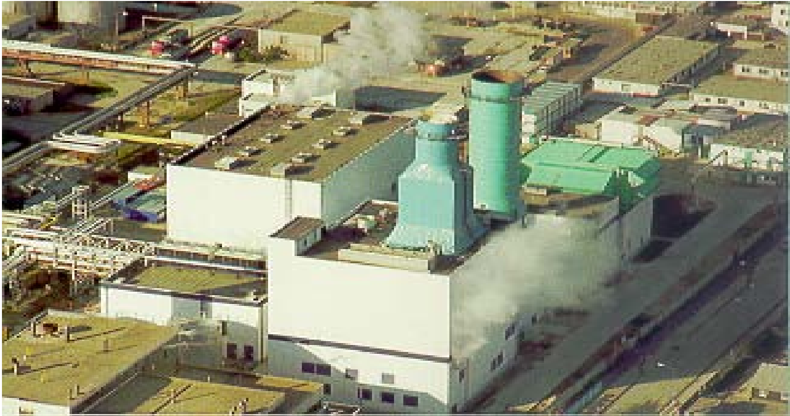
Combined Cycle Power Plant Bratislava, the biggest in Slovakia
