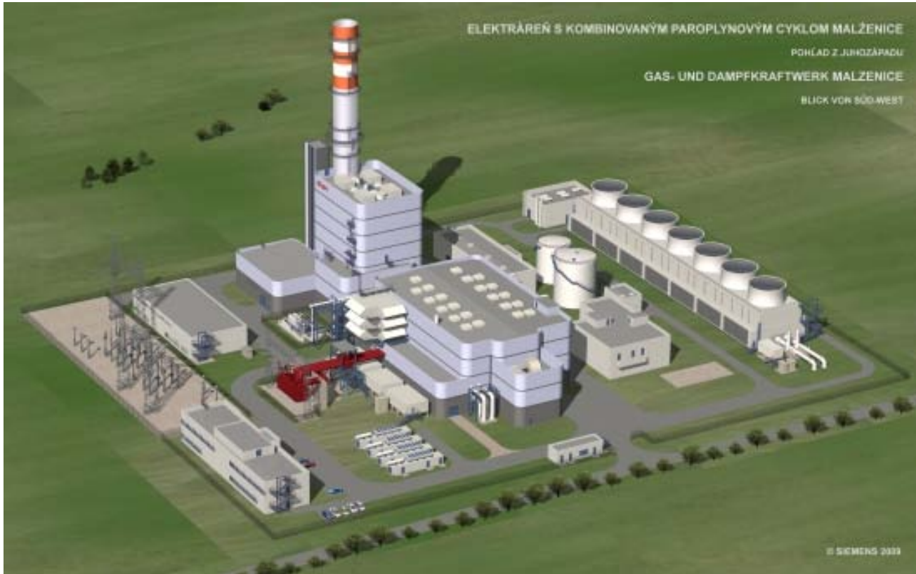
Combined Cycle Power Malzenice, to be commissioned in 2012 Highest thermal efficiency in Europe (59% plus)
