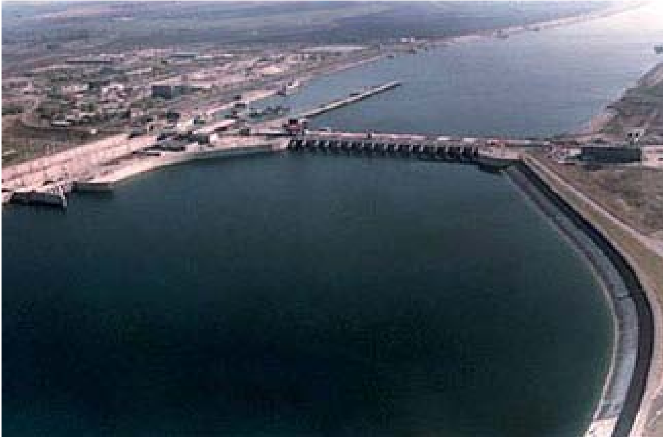
Hydro-electric Plant Gabčíkovo, South-West Slovakia, Capacity 720 MW, the biggest on the river Danube
