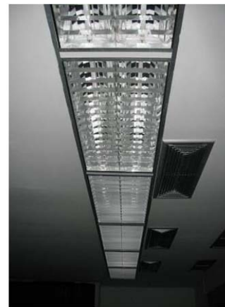
New Fixture-Profile Mirror Louver Type with Aluminum Reflector, T5, 2 x 28 W with Electronic Ballast 550-650 lux
