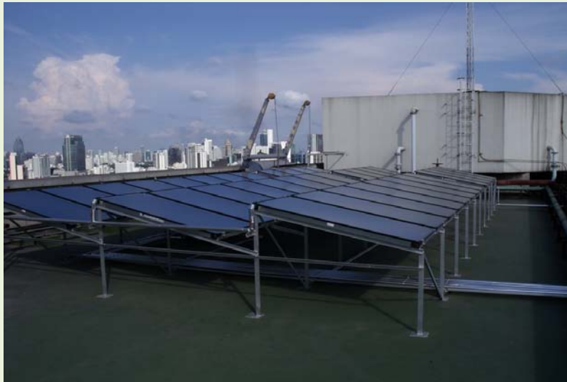
FIGURE B: FLAT PLATE SOLAR COLLECTORS ON THE ROOF TOP OF ROYAL ORCHID SHERATON HOTEL
