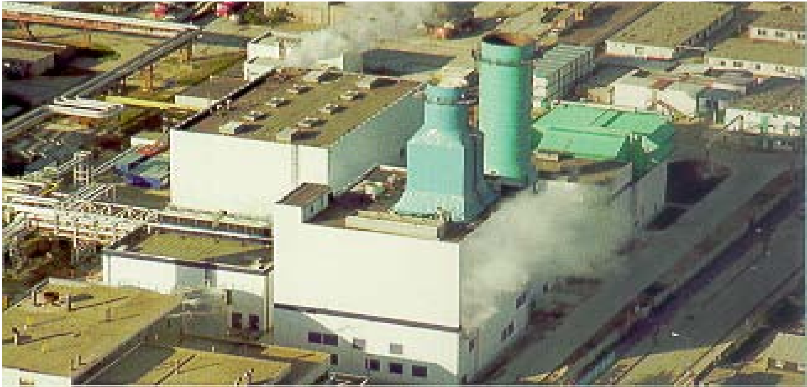
Combined Cycle Power Plant Bratislava, the biggest in Slovakia
